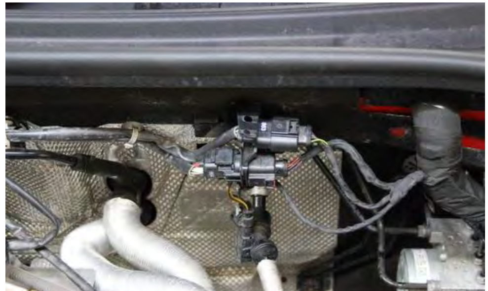
8. We now need to relocate this wiring harness located behind the engine.
